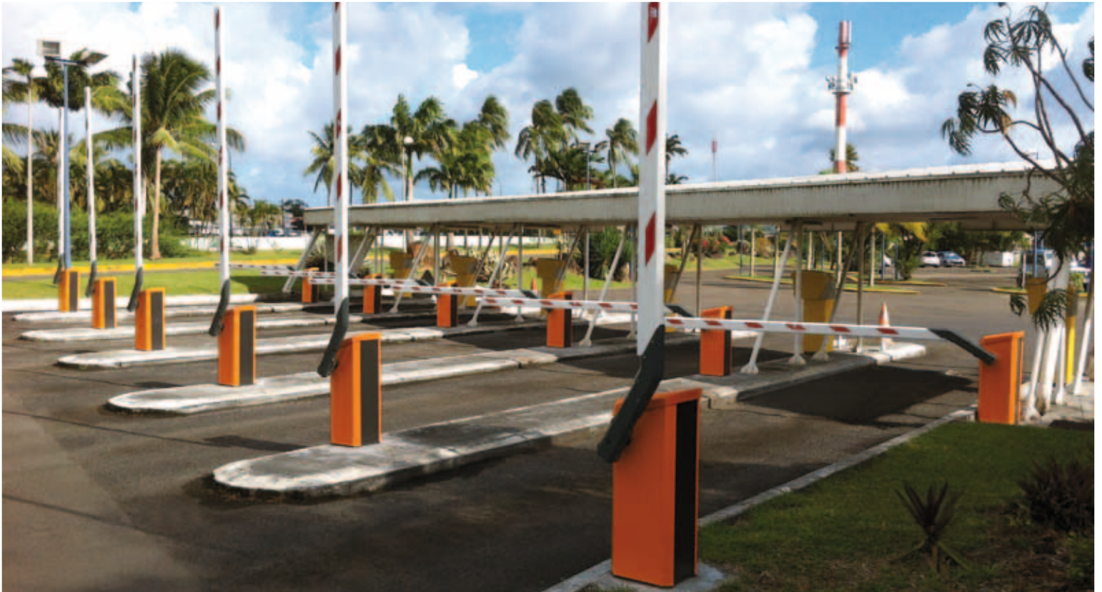
Magnetic Parking barriers as vehicle sluice at Fort-de-France airport (Martinique).
