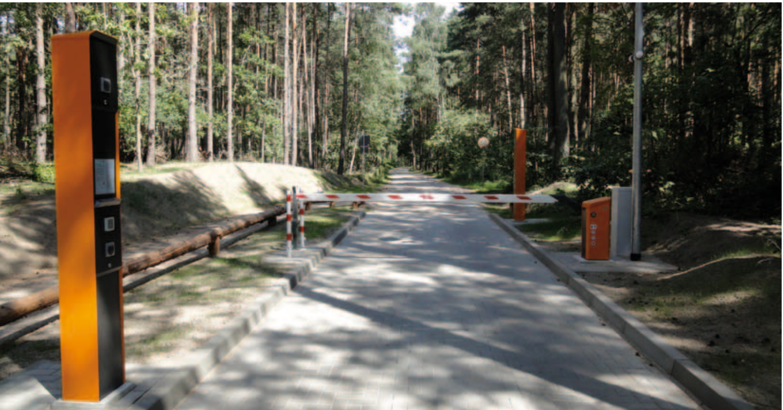
Magnetic.Access barrier in combination with a control column Terminal controls vehicles entering Mueritz National Park.
